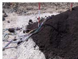
Multi port gas probe units installed in all depth
