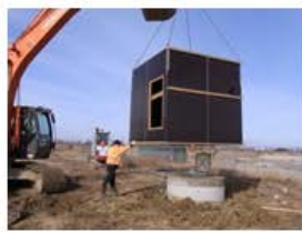
Air tight shed on top of leachate well
