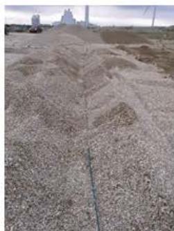
Multi port gas probe units during installation in GDL
