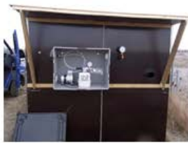
Pump and control unit at well point
