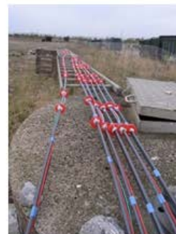
Five multi port gas probes ready for installation in transect
