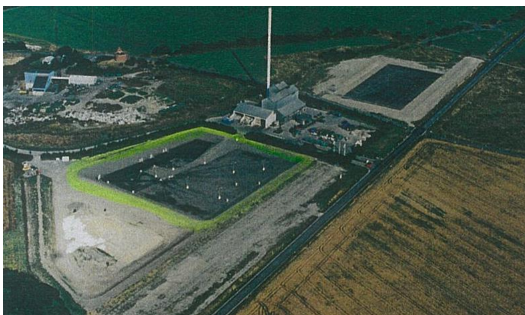
Figure 3.4 Overview of BOFA Landfill.
