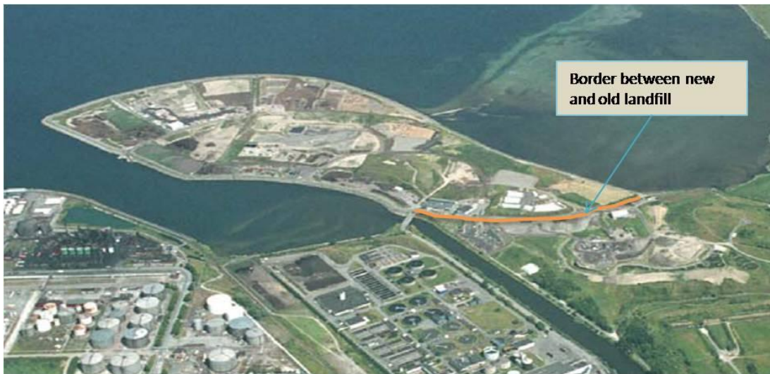
Figure 3.11 Overview of new landfill area at Spillepeng Landfill.
